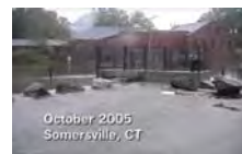
Dams Damaged Due to Flooding From October 2005 Storms
