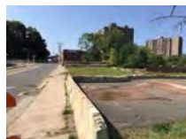
Removal of Structures from Floodplain
