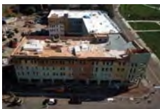
New Elevated Construction
