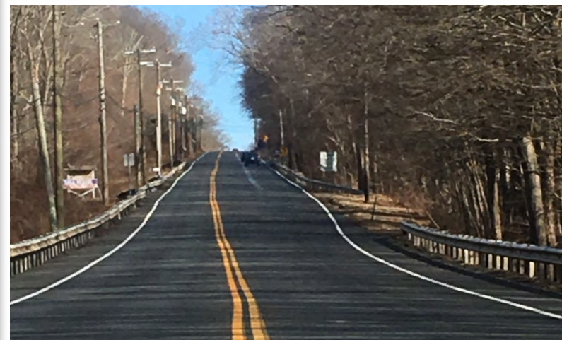
CT-66 Climbing Lanes
