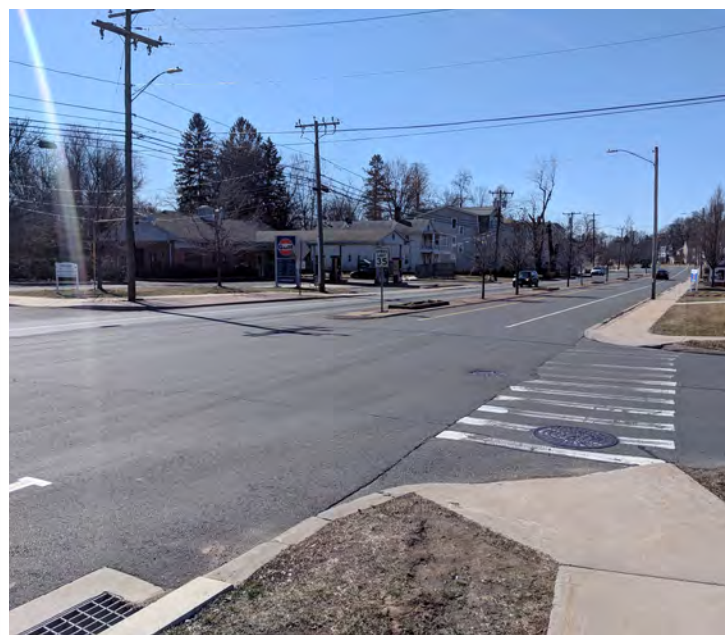
Windsor Avenue and Corey Street
