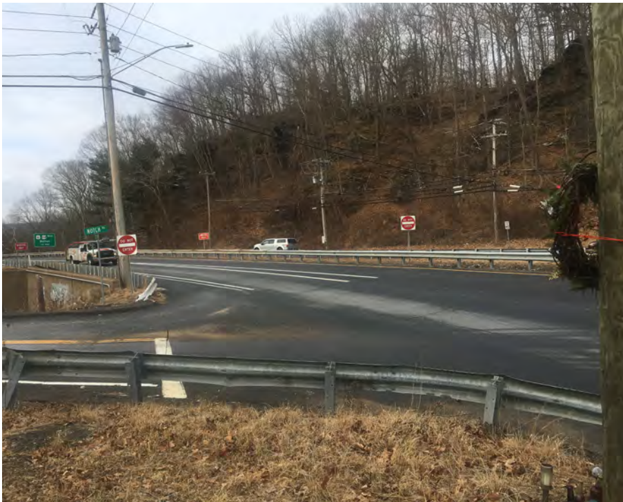
US-6 looking west from Notch Road
