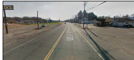
Large Curb Cut & Undefined Driveway
