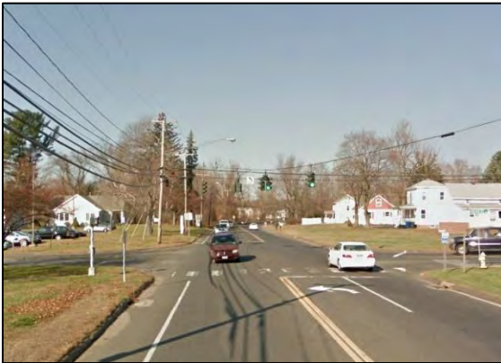
Figure 11: Route 5 NB at Tromley Road and East Windsor High School (Google Street View)
