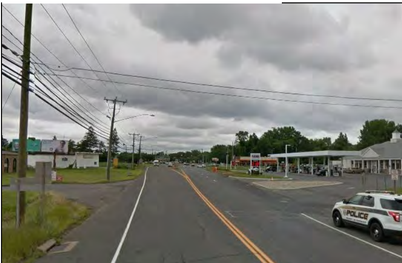
Figure 12: Route 5 NB South of Thompson Road (Google Street View)
