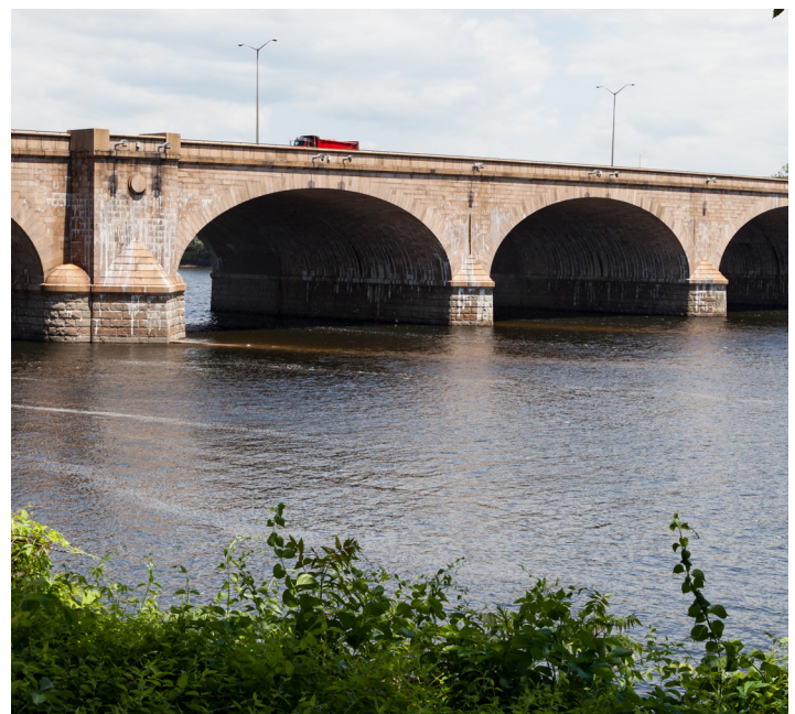
Figure 03.11 — The Bulkley Bridge between Hartford and East Hartford
