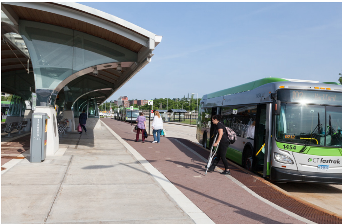
Figure 02.1 – New Britain CTfastrak station
