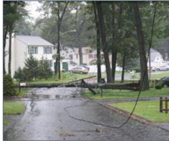
Downed Wires in Enfield after Hurricane Irene
