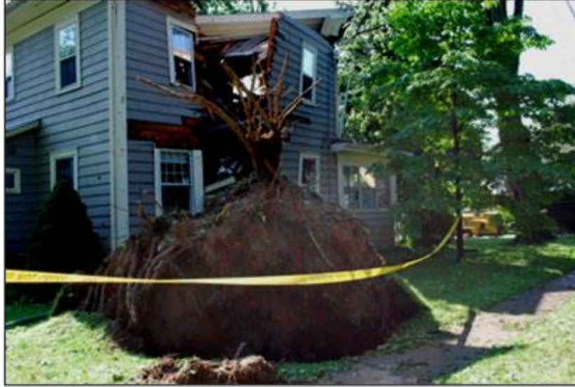
Wethersfield House torn in two by tree toppled during tornado of June 26, 2009
