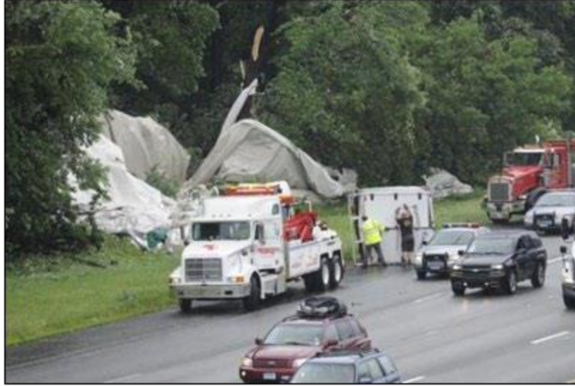
Sports Dome Damage from July 1, 2013 Tornado in East Windsor
