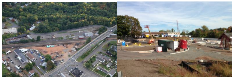
Newington Junction BRT Station
