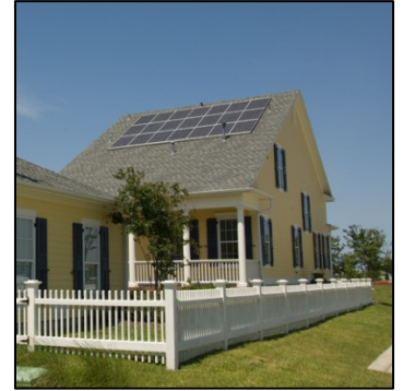
Residential solar panels
