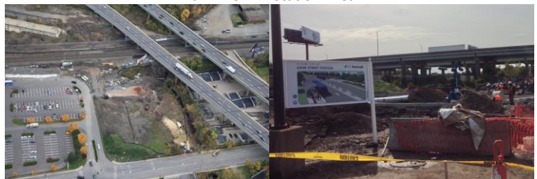
Kane Street BRT Station
