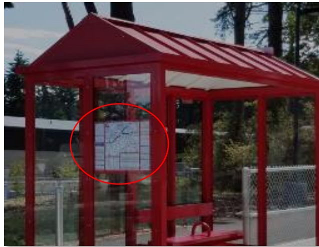
Figure 18: an example of a map case holder in a gable-roofed bus shelter.
