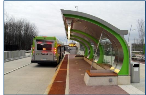
Figure 6: CTfastrak station with curbside tactile warning strips.
