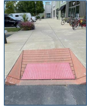
Figure 5: An example of an ADA-Compliant curb ramp at a crossing point.
