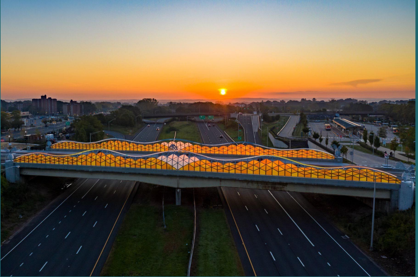
Beehive Bridge, New Britain, CT
