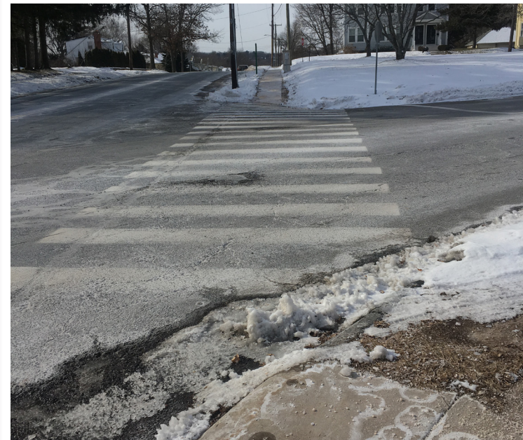
Nott Street at Wolcott Hill Road looking west
