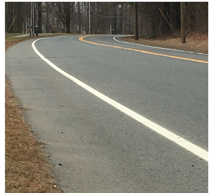
Horizontal curve on CT-168 looking west towards proposed crosswalk site
