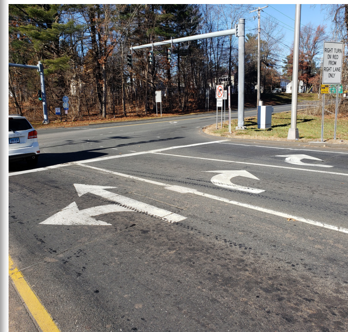
CT-72 ramps at CT-177
