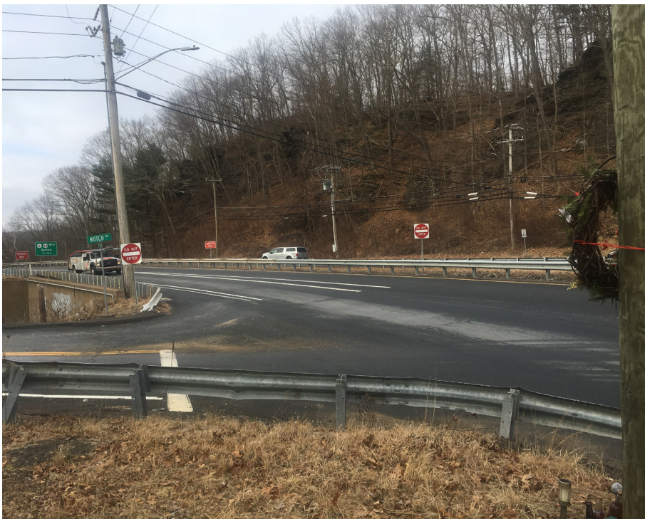
US-6 looking west from Notch Road
