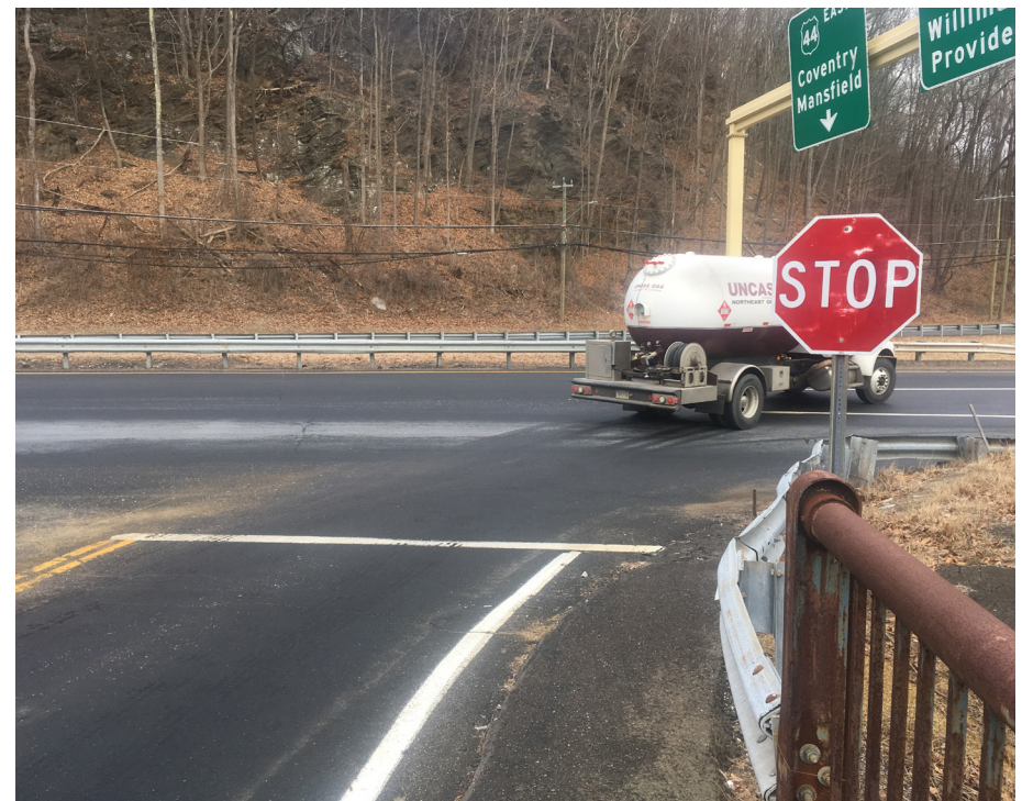
Notch Road and US-6
