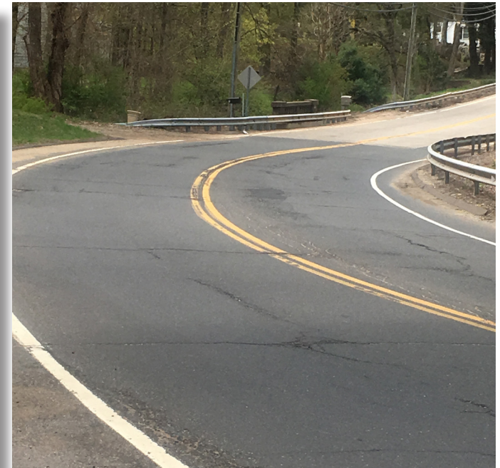
Horizontal curvature along CT-316
