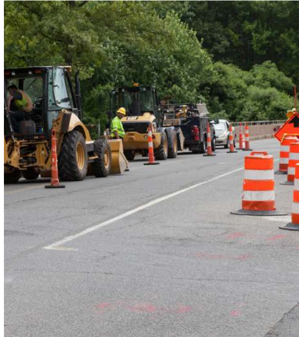
Figure 34: Construction workers repairing a segment of Route 85.
