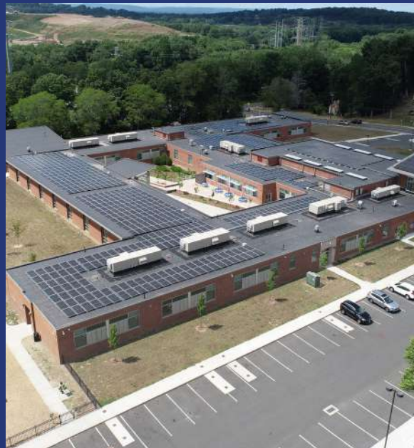
Figure 15: Roof-mounted solar panels at Verplanck Elementary School in Manchester.
