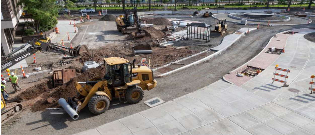
Figure 33: Construction workers building a roundabout in New Britain.
