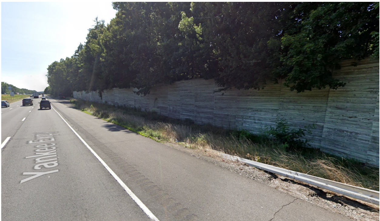
Figure 3 – Noise barrier separated from I-84 westbound by grass buffer
