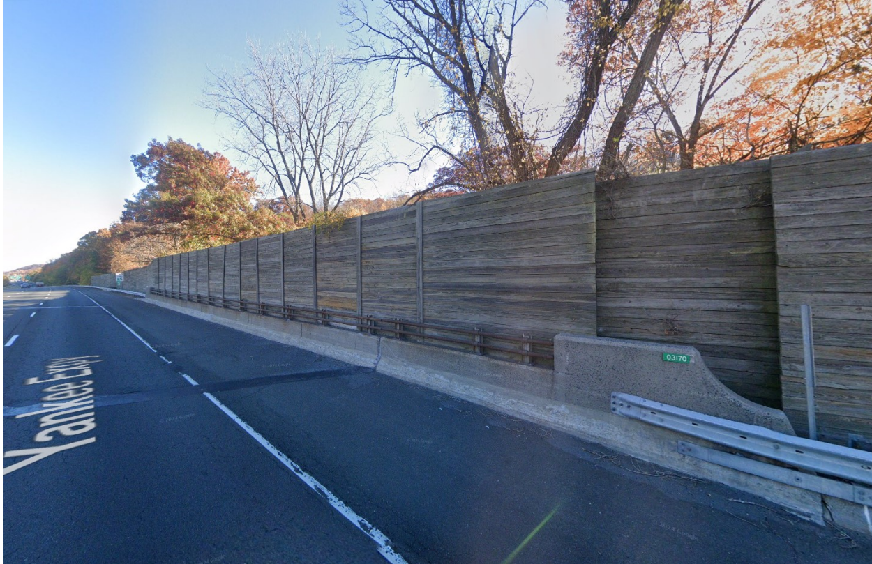
Figure 4 - Structure mounted noise barrier wall on bridge 03170
