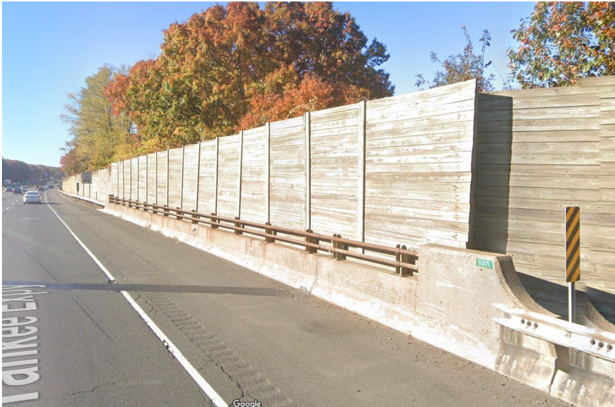
Figure 2 - Structure mounted noise barrier wall on bridge 03171
