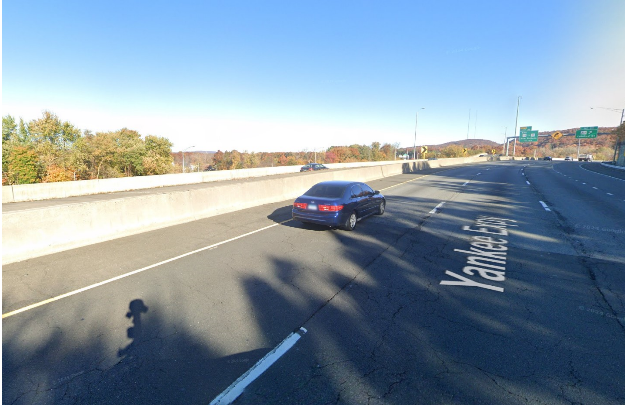
Figure 7 - Concrete barrier dividing the mainline of I-84 eastbound with ramp 84-E-813
