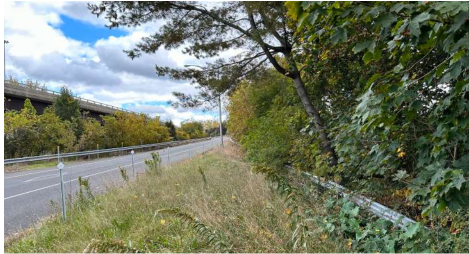
View of the I-84 eastbound entrance ramp from Mercer Avenue and Silver Lane
